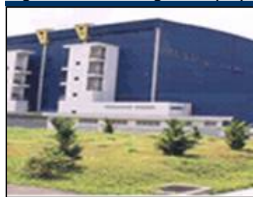
Figure 24: Plentong Plant (JB)
